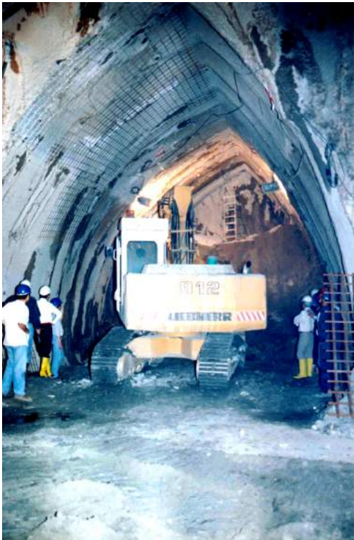
Figure 25: Twin side drift and central pillar excavation method. Temporary support consists of double wire mesh reinforced 250 - 300 mm thick shotcrete shells with embedded lattice girders or HEB 160 steel sets at 0.75 - 1 m spacing.
