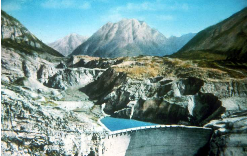
Figure 2b: During the filling of the Vajont reservoir the toe of the slope on Mount Toc was submerged and this precipitated a slide. The mound of debris from the slide is visible in the central part of the photograph. The very rapid descent of the slide material displaced the water in the reservoir causing a 100 m high wave to overtop the dam wall. The dam itself, visible in the foreground, was largely undamaged.
