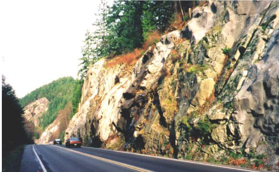
Figure 11: The Argillite Cut on Highway 99 in British Columbia, Canada.
