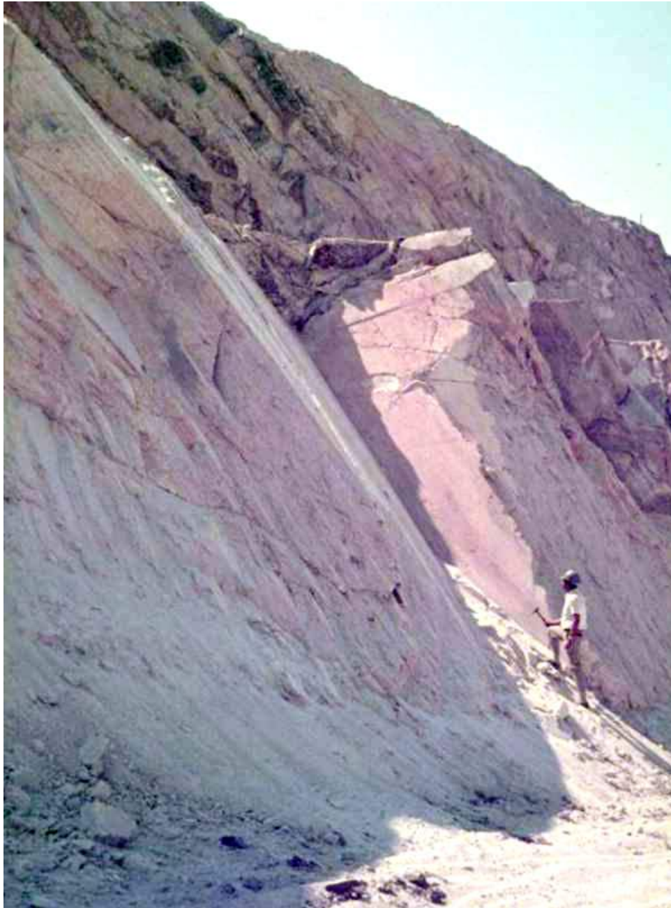
Figure 4: A wedge failure controlled by intersecting structural features in the rock mass forming the bench of an open pit mine.
