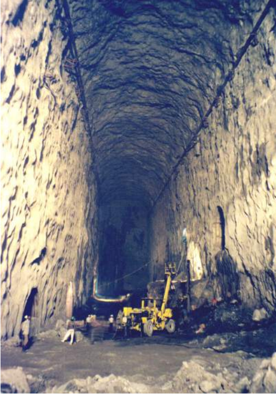
Figure 22: Partially completed 20 m span, 42.5 m high underground powerhouse cavern of the Nathpa Jhakri Hydroelectric Project in Himachel Pradesh, India. The cavern is approximately 300 m below the surface.
